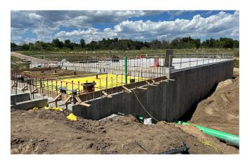
To address the harsh conditions within the lift station, Xypex Bio-San was incorporated into the concrete mix, providing integral protection against microbial-induced corrosion (MIC) caused by high levels of hydrogen sulfide (H2S). Its advanced crystalline technology enables self-healing of micro-cracks and resistance to hydrostatic pressure, ensuring long-term impermeability and structural integrity.
